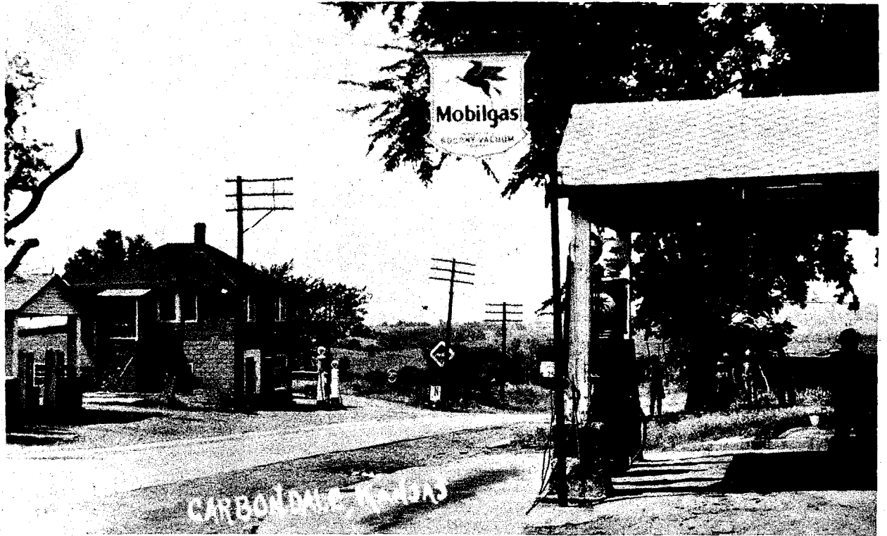
Finished highway 75 into Carbondale 1928. Isreal Shepard's filling station to right, Romine Garage to left.
