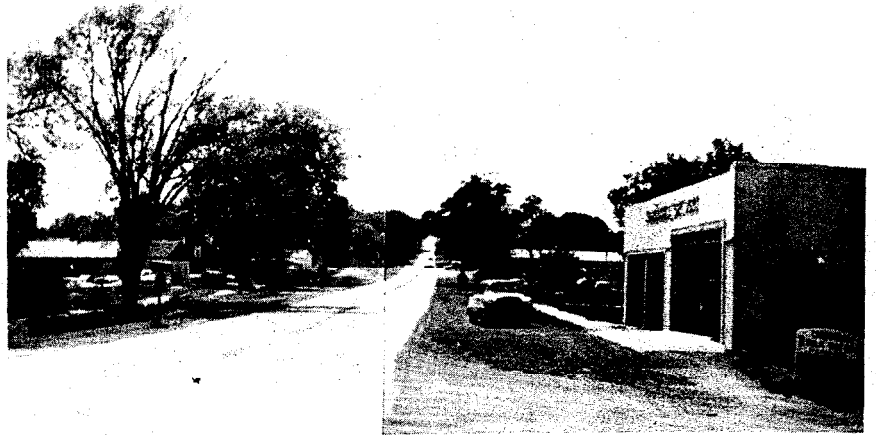
Carbondale 1972, 2nd Street looking west
