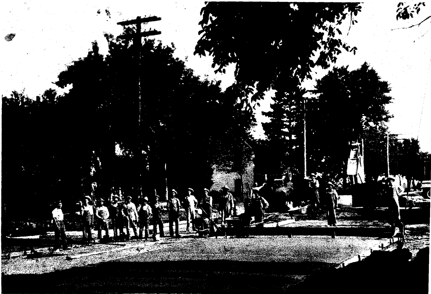
The Highway 75 Insertion to downtown Carbondale Work Crew built in 1926.
