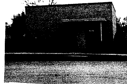
Southwestern Bell Telephone office
