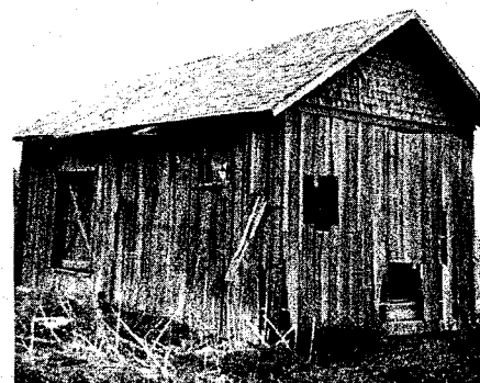
Old Carbon Hill Depot 1 1/2 mile Southeast of Carbondale. Built 100 years ago.
